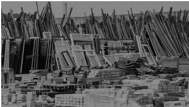
Fig. 3.6 Salvaged products recovered in a process of selective demolition. Source: Rinnovabili.it, 2017. Available at: http://www.rinnovabili.it/riciclo/riciclo-materiali-edili-costruzioni/ .
